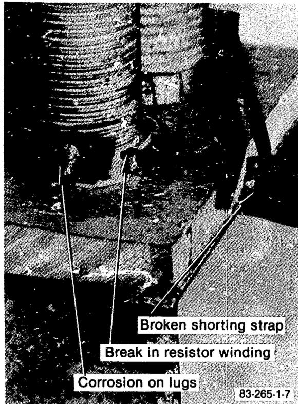
Figure 18. Insulation corrosion and winding breakage in the polar crane.
