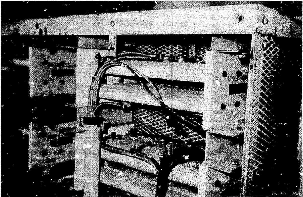
Figure 17. Typical polar crane resistor bank installation.
